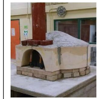
5) Fill side wall cores completely with insulating castable. Parge entire oven dome with insulating castable refractory at least 2" thick.
