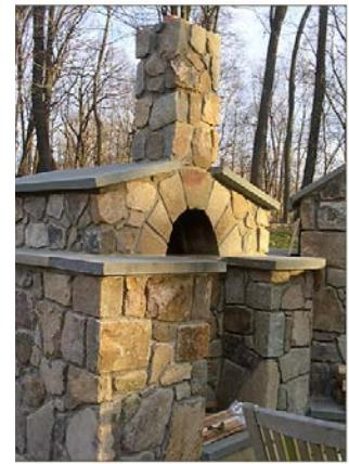
7) The 4"x8" flue liner should be enclosed within a chimney with walls at least 4" thick of solid masonry. If the chimney is inside a house it must conform to all applicable codes dealing with clearance to combustibles and height above the roof. If the oven is outside the flue need only be enclosed in masonry as high as is desired and clear of combustibles.
