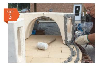
Lay out a 36" circle on oven floor and set the 2-piece entrance tunnel and two sidewalls using HeatStop II refractory mortar.
