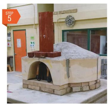
Parge dome with insulating refractory concrete at least 2" thick. Fill cores of side sections and entrance sections with insulating refractory concrete.
