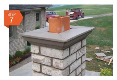
The 4" x 8" flue liner should be enclosed within a chimney with walls at least 4" thick of solid masonry. If the chimney is inside a house, it must conform to all applicable codes dealing with clearance to combustibles and height above the roof. If the oven is outside, the flue need only be enclosed in masonry as high as is desired and clear of combustibles.
