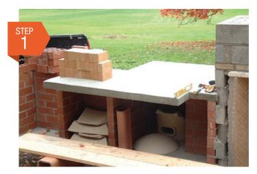
Build masonry base at least 52" wide by 64" deep, and 38" high for a finished oven floor 42" above the kitchen floor or ground.
