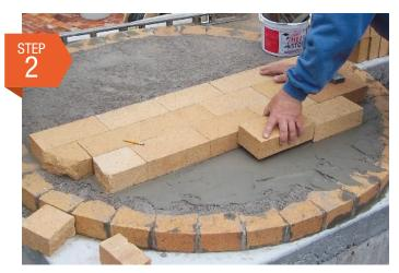
Cast a 2" thick layer of insulating refractory concrete on top of the base and set the firebrick oven floor directly on the insulating refractory concrete.
