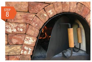
An entrance cover for the oven entrance is provided to help keep the oven warm. It can be propped up slightly (to provide combustion air) at the outside of the entrance when a fire is burning in the oven and can be pushed in farther to close off the flue to keep the oven warm longer after the fire has burned out.
