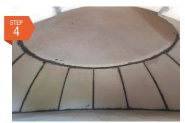
Set the 32" oven dome, and the first flue tile all in Heatstop II refractory mortar.
