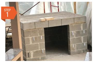
Build masonry base at least 67" wide by 67" deep, and 38" high for a
