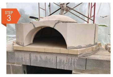
Set wall sections (8 pcs) and the entrance tunnel (3 pcs) as shown using HeatStop II refractory mortar.
