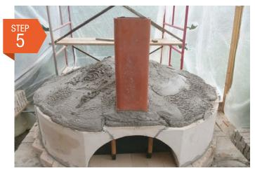
Parge dome with insulating refractory concrete at least 2" thick. Fill cores of side sections and entrance sections with insulating concrete.
