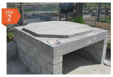
Cast a 2" thick layer of insulating refractory concrete on top of the base and set the firebrick oven floor directly on the insulating refractory concrete. Oven outside diameter is 65".
