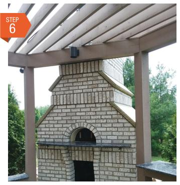
The oven can be stuccoed, plastered or finished with any non-combustible masonry material such as tile, brick or stone.
